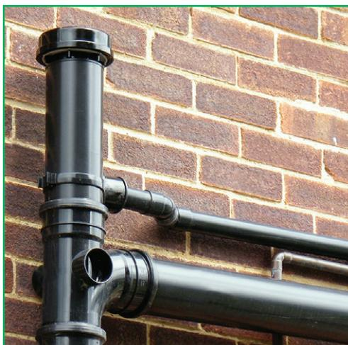
Document H Clause 1.31 states that "Ventilating pipes open to outside air should finish at least 900mm above any opening into the building within 3 metres". This new development by FloPlast, of an External Air Admittance Valve, will allow the installation of an external soil pipe within 3 metres of any opening and terminate at the same height as if it were installed internally, ie. 200mm (minimum) above the highest wet entry point to the soil vent pipe. See diagram below.
