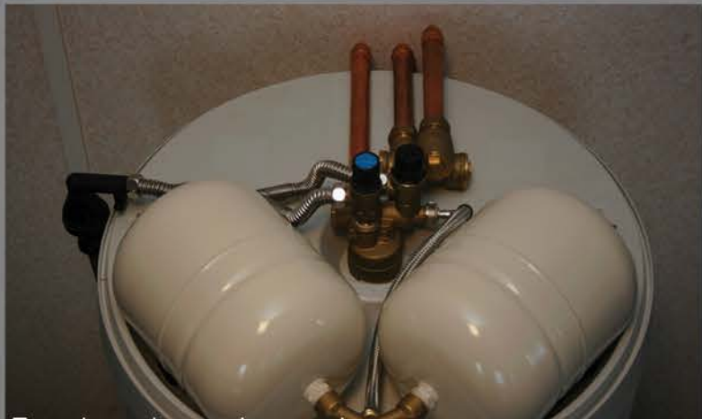
Top valve and expansion vessels
